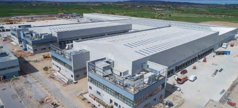
UPS Warehouse, Essex
