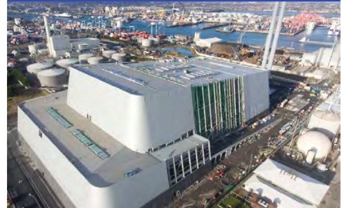
Covanta Power Station, Dublin
