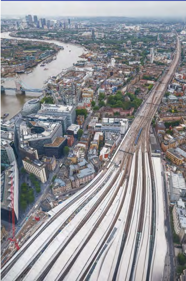
London Bridge Station Canopies
