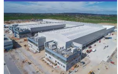
Industrial and distribution
