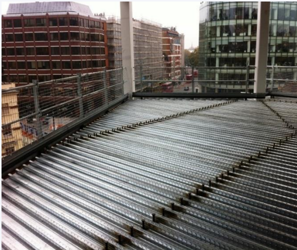
Metal decking and studs
