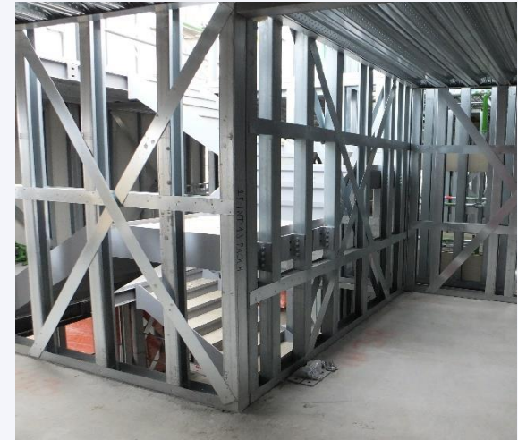
Load bearing framing
