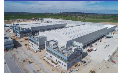
Industrial and distribution
