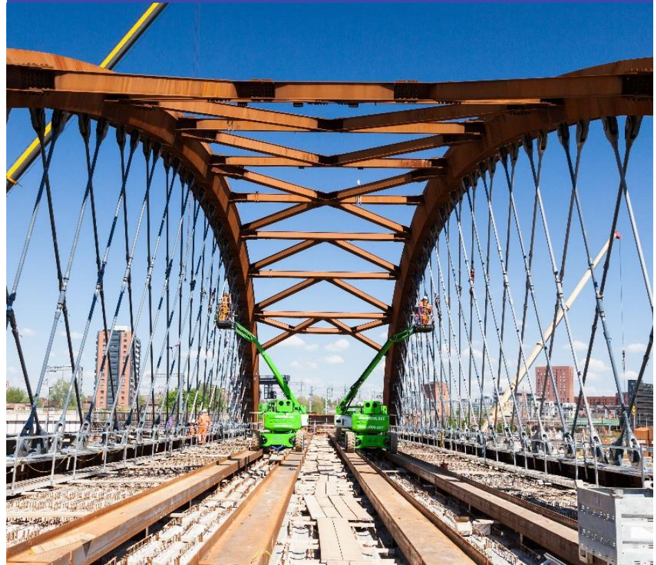
Ordsall Chord, Greater Manchester
