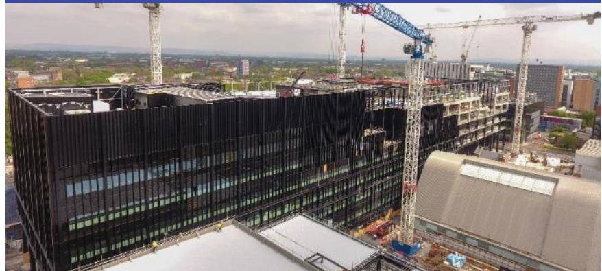
Manchester Engineering Campus Development
